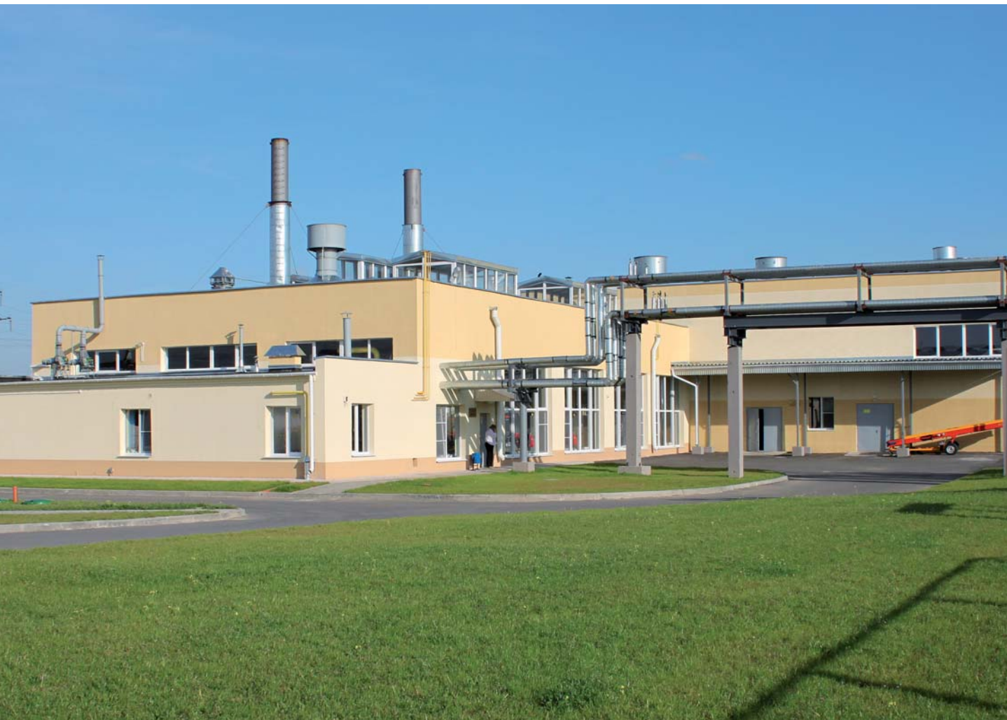
SSAO Servolux, Litauen, 3 St. Vitomax 200-HS 4 t/h; 13 bar.
