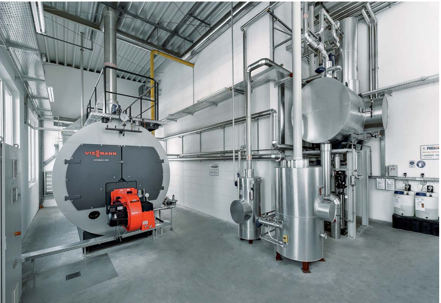
StoVerotec, Deutschland, Vitomax 200-HS, 4t/h, 16 bar
