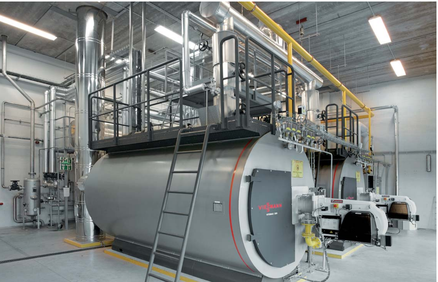
Vitomax 200-HS; 3,8t/h, 13 bar in Belgien
