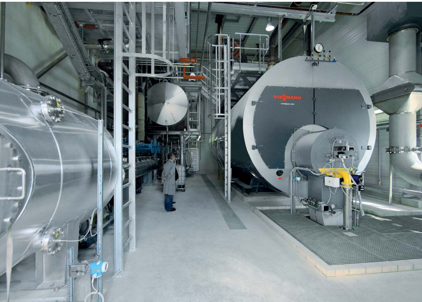
Vitomax 200-HS, 26 t/h, Austria
