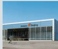
Ameco A380 Hangar Peking, China
